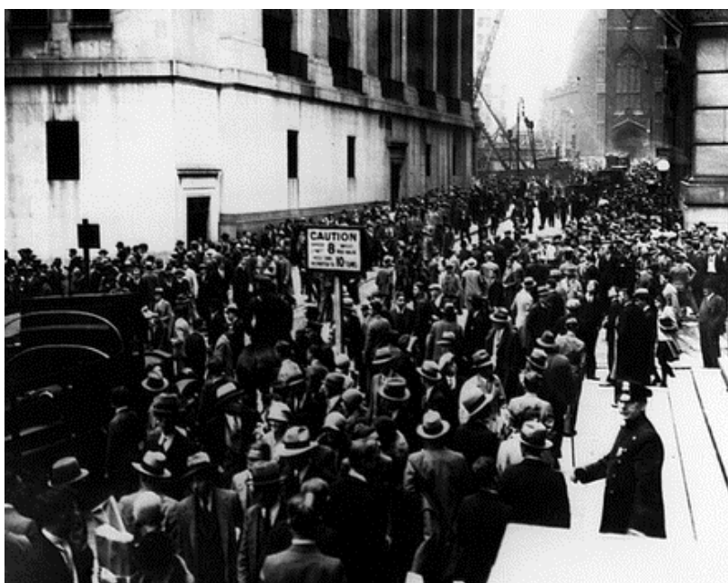
Crack do 29, NIC.
