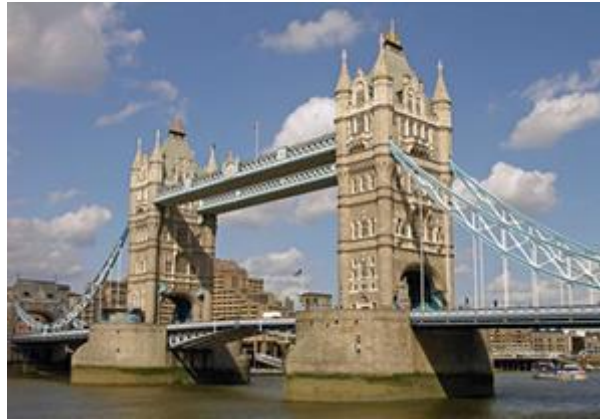
Tower Bridge (Londres)
