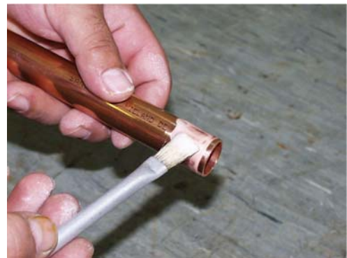
4. Apply the soldering flux on the pipe
